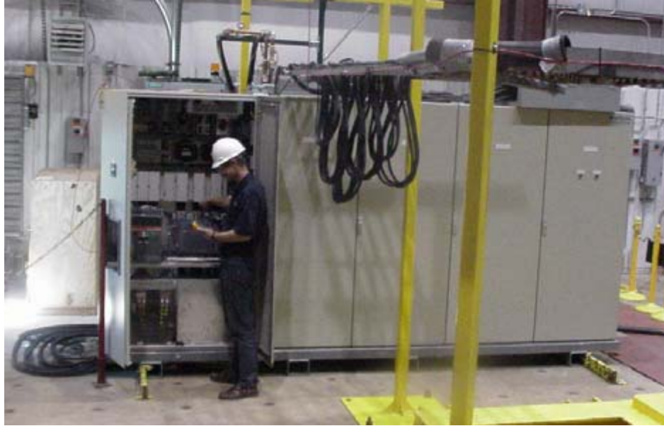
Figure 5-5. The power electronics connected to the generator via overhead trays, and connected to the grid via trays on the floor.
