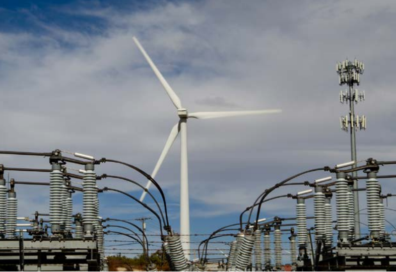
Accelerated growth in wind and solar generation will require a corresponding supply of step-up transformers. Photos from Getty Images, top: 1406020186, bottom: 1284482079
