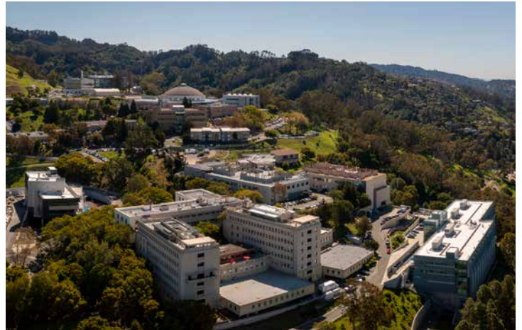
Tianzhen Hong, Kaiyu Sun, and Jeetika Malik are working towards the commercialization of a web-based data and computing platform providing energy modeling, benchmarking, and performance visualization of a city's building stock. Photo from LBNL
